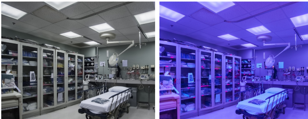
Images of white antimicrobial and architecture lighting (left) versus violet enhanced antimicrobial only (right), courtesy of Results with VioSafe™ in Active Trauma Room at Samaritan Hospital, Troy, NY
